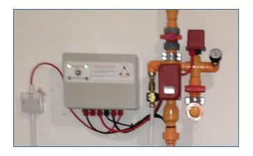
The photograph above shows the controller, (measuring 300mm by 220mm) alongside the sprinkler controls, (measuring 300mm by 525mm). These items are typically mounted above the water tank but this is not a requirement.
